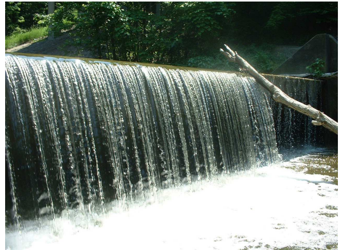
East Branch Dam
