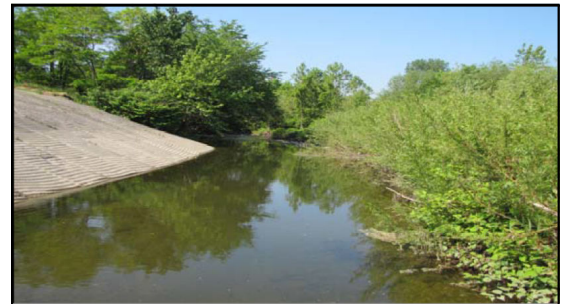
Alen Michael's donation will help protect and restore part of Euclid Creek, pictured above.
