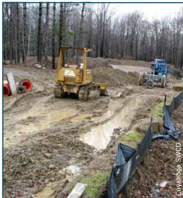
Wet construction conditions contributes to increased compaction and decreased infiltration.
