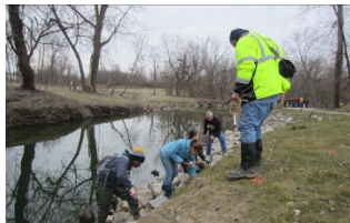
Volunteers planting live stakes along a streambank to help protect the slope (left) and trees installed on the wetland (right)
