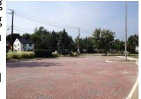
South Euclid City Hall's new permeable parking lot
