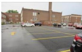
Shore Cultural Center's permeable parking (left) installed only in the parking spots as is evident from infiltration after recent rain. Rain flowing over traditional asphalt flows into bioretention cell for infiltration (right).
