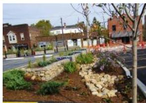
The 'Azure Stained Glass' parking lot at E. 156th and Waterloo was retrofitted with bioretention to hold and filter pollutants from the surrounding parking lot (left). Closeup of colored blue glass used in the design (right).
