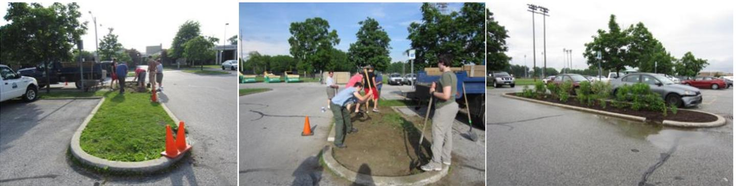
Median before installation (left photo); soil excavation to install more infiltrative soil (center); and completed rain garden (right)
