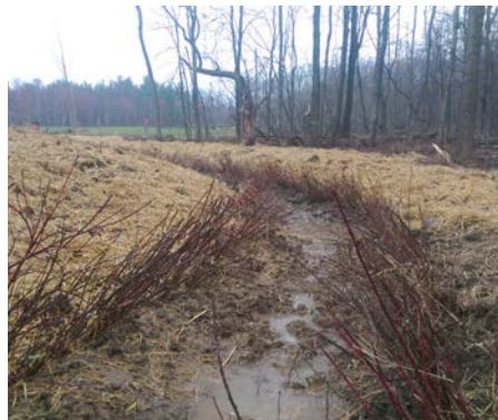
Dogwood planting during construction
