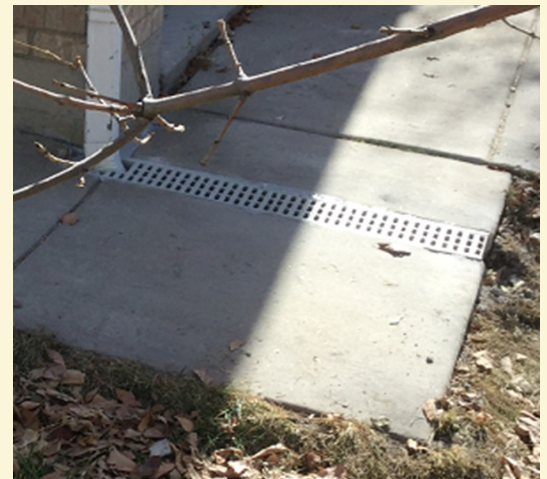
This sidewalk was cut to connect a downspout to a rain garden. This is an option to consider.
