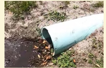
An inflow pipe with debris. Photo credit: Aqua Cleaning
