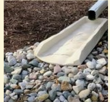
A splash block can also lead water away from a foundation. Photo credit: GreyDock
