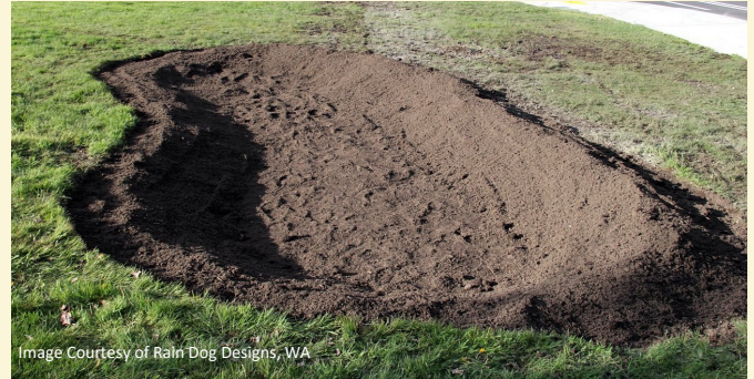
A dug rain garden basin with berm to the right.
